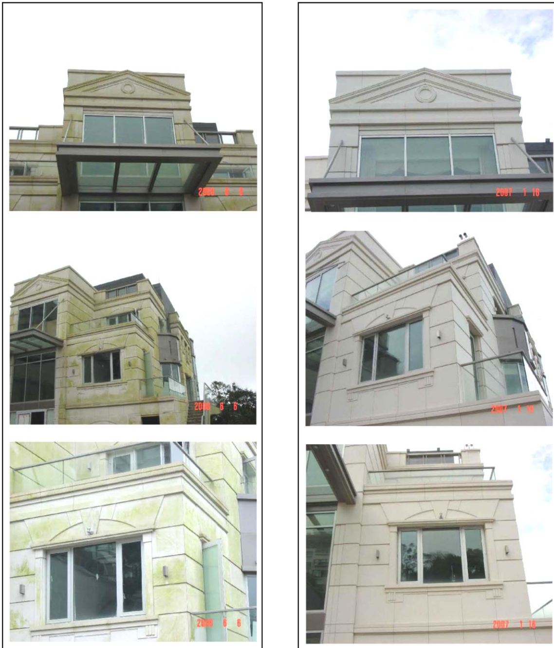
Fig 12: The difference between using ordinary paints and paints made by nanotechnology and the impact of environmental factors after 224 days
