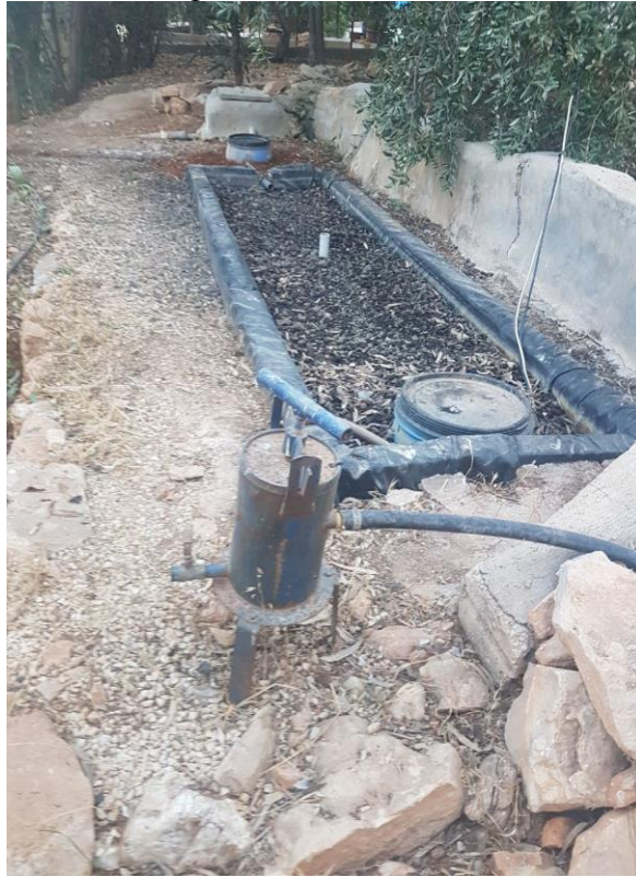
Fig (3): Greywater Station
