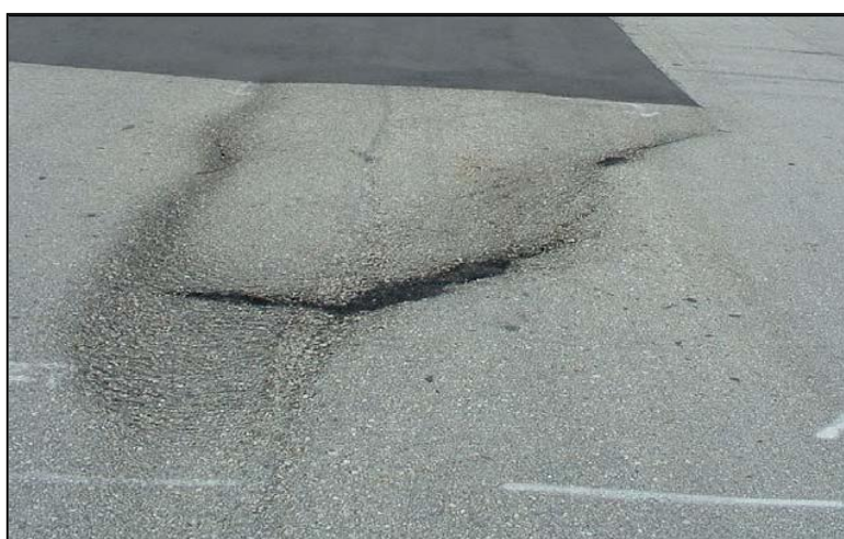
Figure 1.1 : Slippage Failure Due to Poor Bond between HMA Layers.
