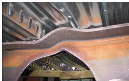
Figure 1. Vierendeel Mechanisms [1]
