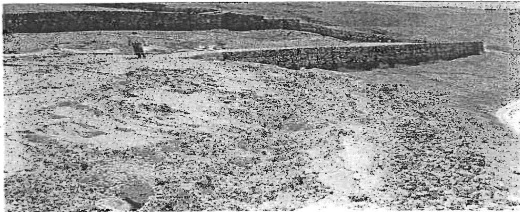
Figure 9. February 23, 1997 landslide at WESTP project, (a) the dislocation and separation of the gabion wall in the middle of the slide, (b) the standing undisturbed gabion adjacent to the displaced one with a dislocation of about 6 to 9m at the toe of the slide.
