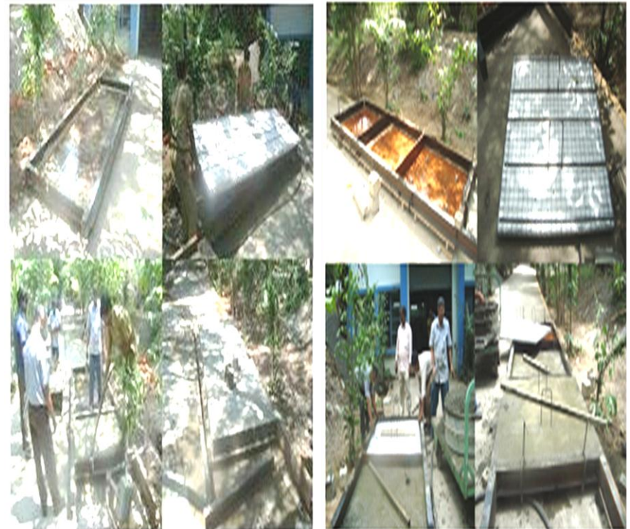
Casting of 3D sandwich wall panel
