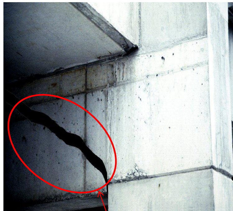
Shear failure
