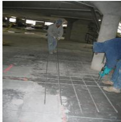
Fig.: Near Surface Mounted (NSM) Technique
