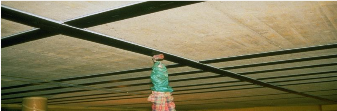
Fig.: Externally bonded reinforcement (EBR) Technique
