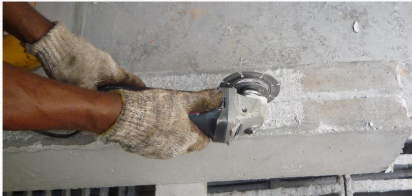
Fig. Cutting of the groove and cleaning the groove by air jet
