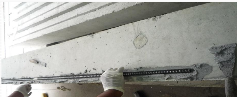
Fig. Insert the bar and fill up the groove after insert the bar
