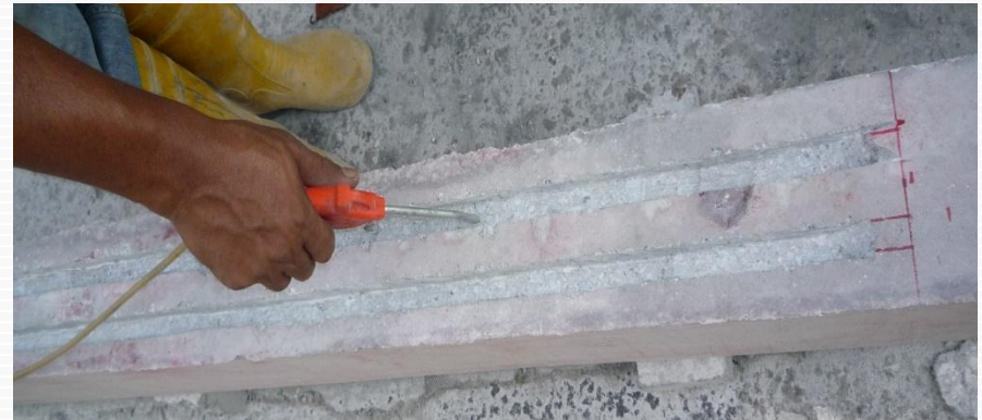
Fig. Cutting of the groove and cleaning the groove by air jet
