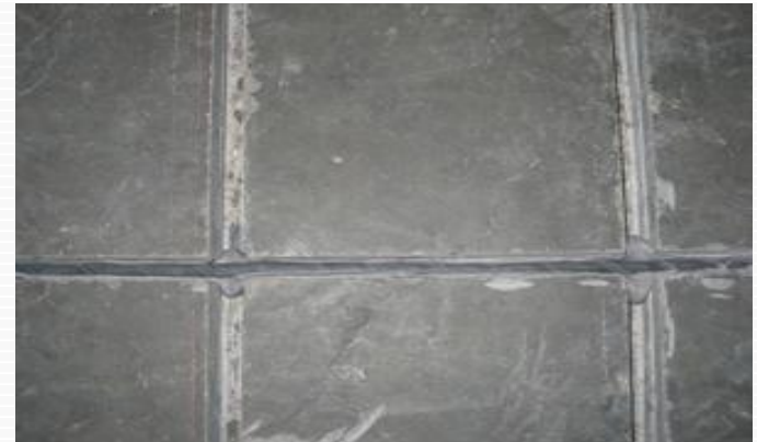
Fig.: Externally bonded reinforcement (EBR) Technique
