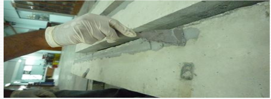
Fig. Insert the bar and fill up the groove after insert the bar
