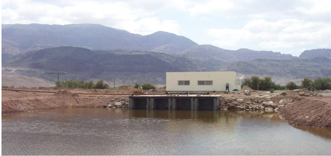
Photo (2): Collection Lagoon For Drainage Water At Sammar Site
