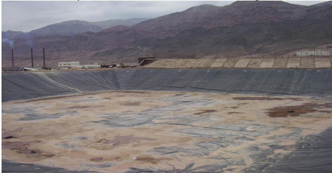
Photo (3): Refinery Collection Pond For Sub-Surface Drainage Water
